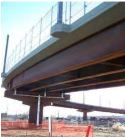
Figura 1.7. Puente sobre vigas I curvas de acero ([http://denverurbanism.com/wp-content/uploads/2011/12/2011\\_12\\_30\\_CMLBridge05.jpg](http://denverurbanism.com/wp-content/uploads/2011/12/2011_12_30_CMLBridge05.jpg)).
