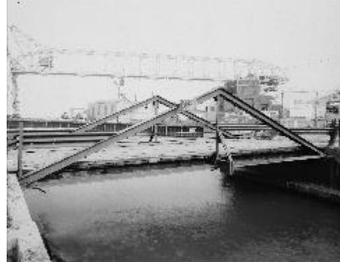
Figura 1.2. Puente viga tipo King Post, 1920 ([https://upload.wikimedia.org/wikipedia/commons/4/4b/King\\_post\\_truss.jpg](https://upload.wikimedia.org/wikipedia/commons/4/4b/King_post_truss.jpg)).
