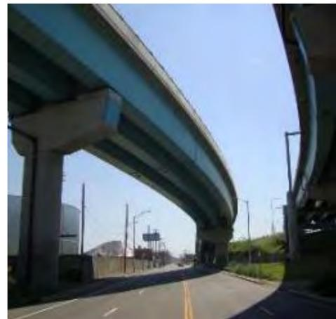
Figura 1.8. Puente sobre vigas-cajón curvas de acero ([http://alwayscivil.blogspot.com/2009\\_08\\_23\\_archive.html](http://alwayscivil.blogspot.com/2009_08_23_archive.html)).
