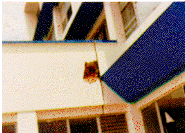
Figura 2.55 Hospital de Tena
