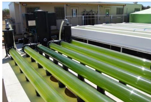
Figura 2.5 Fotobiorreactor tubular de tubos horizontales paralelos (STELR Project, 2010)
