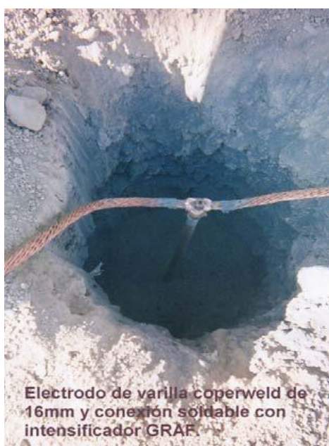
Figura 4.2 Varilla Copperweld
